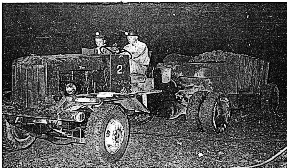
FIGURE 4 A 10 TON DIESEL TRUCK-TRAILER
